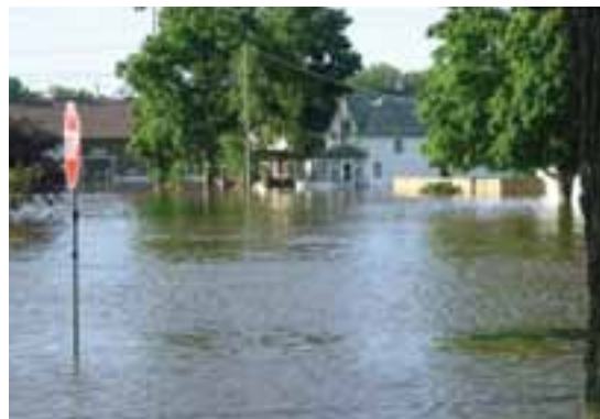
Three blocks of Vinton, Iowa, flooded in 2008, including the electrical plant.
